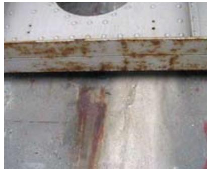
moisture through the coating, causing active corrosion of the substrate *long before* the protective coating fails.
