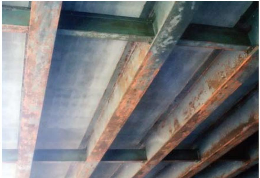
**ABOVE** ▲ Surface contamination by soluble salts has long been an issue for the corrosion industry. Lead-based paints used to be the first line of defense. A unique property of lead is that it reacts with soluble salts to form insoluble salts, thereby preventing those salts from causing or increasing corrosivity. But, of course, lead-based paints resulted in toxicity problems that outweighed their usefulness as anti-corrosives.
