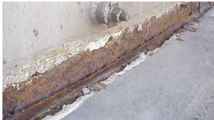
cause osmotic blistering of concrete coatings. These salt contaminants can also be introduced onto a concrete surface when etched by or exposed to hydrochloric or sulfuric acid.
