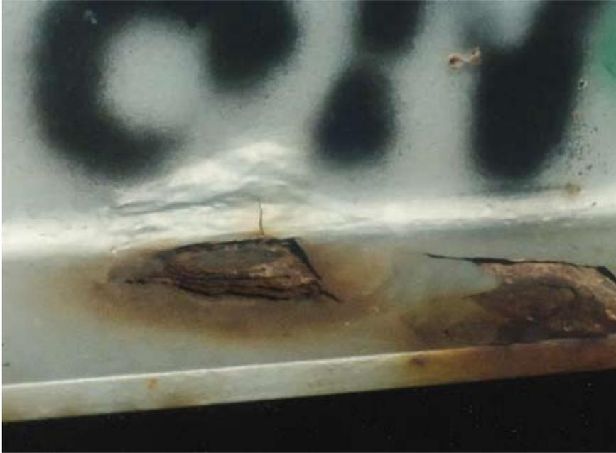
**LEFT** ◀ All liquid-applied coatings are moisture-vapor permeable and will allow the salt on a substrate to “draw” moisture through the coating, causing the active corrosion of the substrate long before the coating fails.
