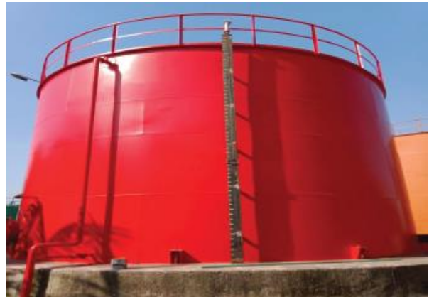
Application of PU topcoat 50 – 60 \mu\text{m} DFT & delivery to the client CLC POWER in November 2020
