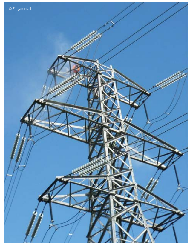
Figure 2 - Vapour-blasting an electricity pylon.
