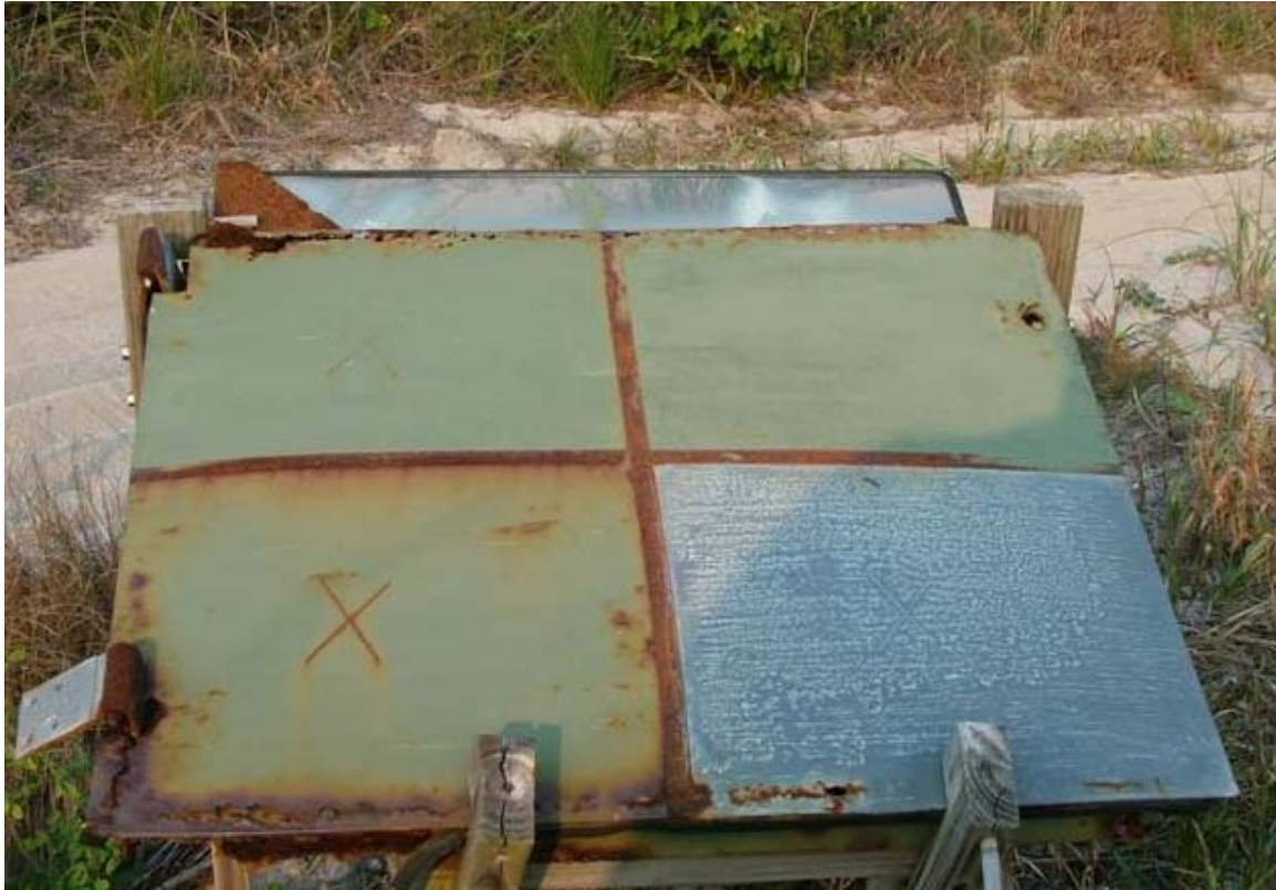
Figure 2. 5-Ton Truck Door at KSC.
